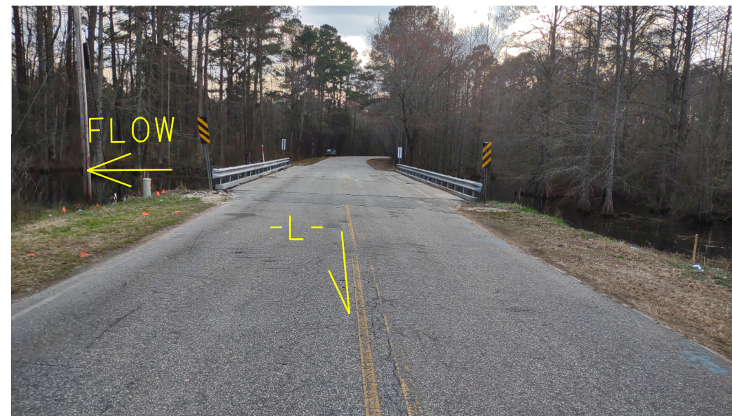
PHOTO #3: BRIDGE NO. 015 AT END BENT 2 LOOKING WEST (DOWNSTATION)
