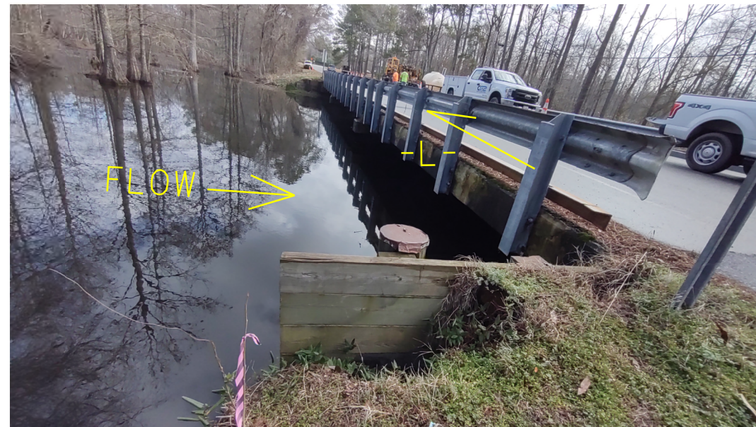
PHOTO #1: BRIDGE NO. 015 AT END BENT 1 (LT) LOOKING EAST (UPSTATION)
