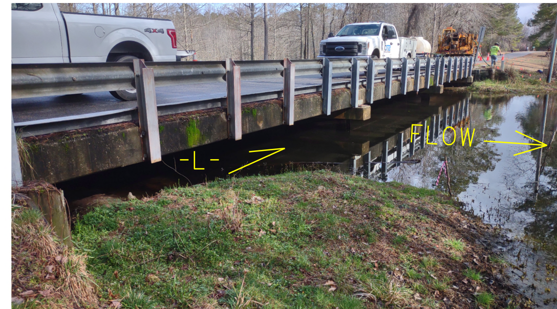
PHOTO #2: BRIDGE NO. 015 AT END BENT 1 (RT) LOOKING EAST (UPSTATION)
